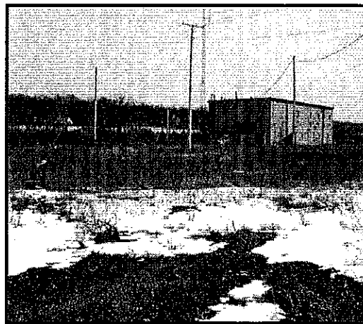
View of the existing on-site office building to be demolished during the site clean-up.
